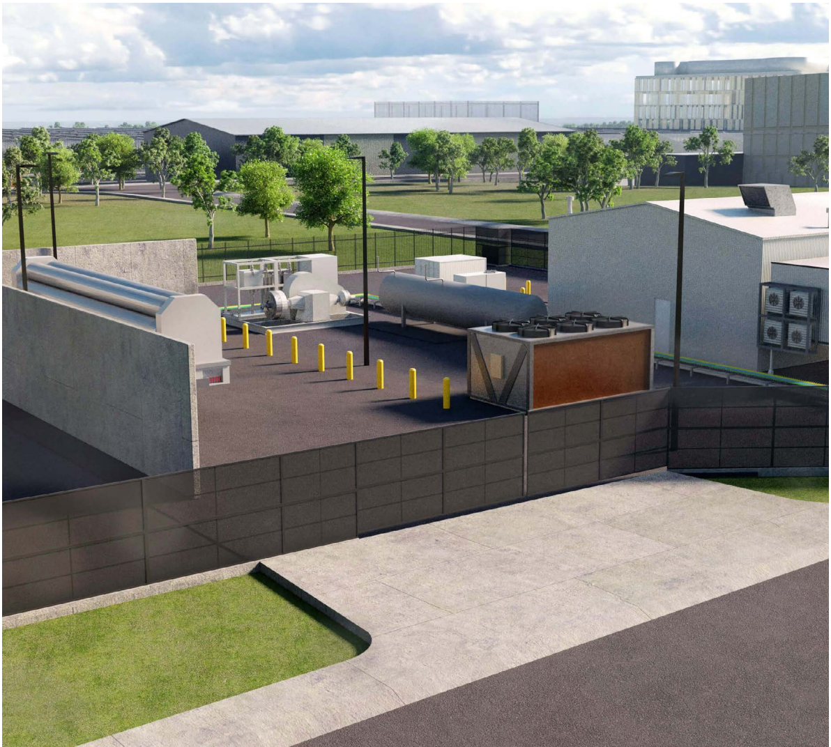
Artist impression of AGIG’s proposed Hydrogen Park SA (HyP SA), featuring a 1.25 MW electrolyser capable of supplementing electricity grids with power generated from renewable sources.
